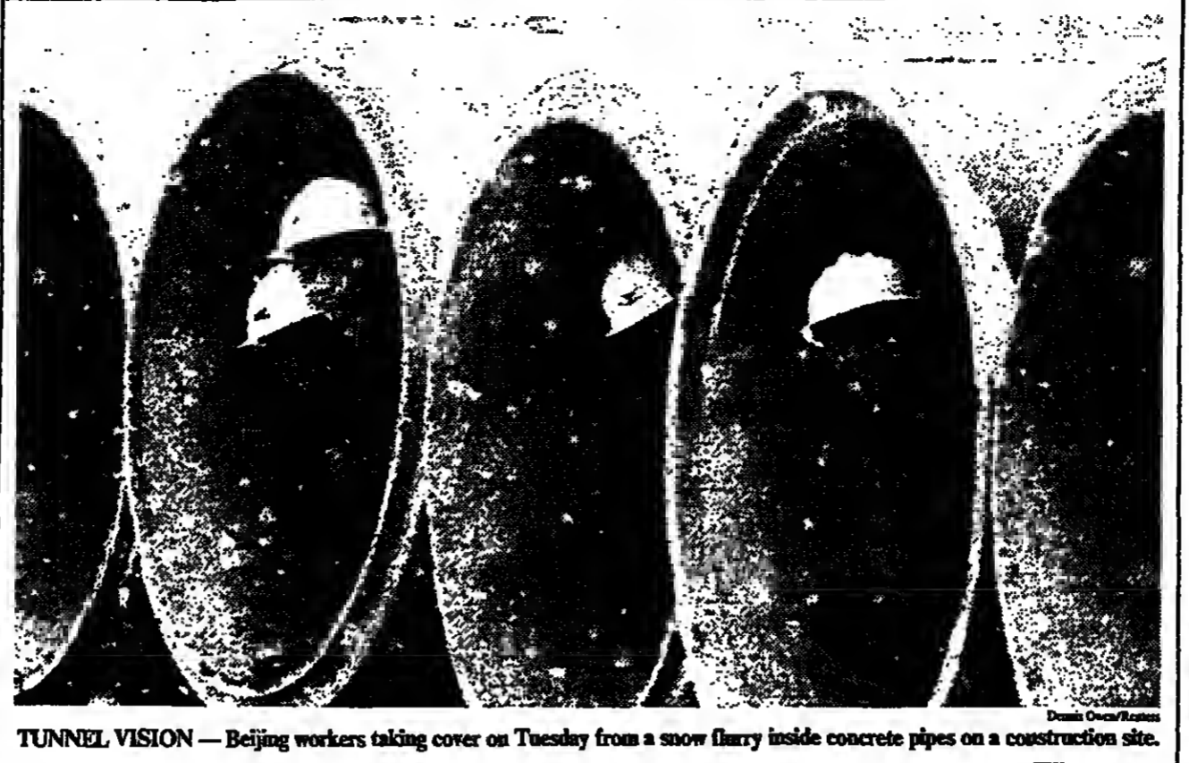
TUNNEL VISION — Beijing workers taking cover on Tuesday from a snow flurry inside concrete pipes on a construction site.
